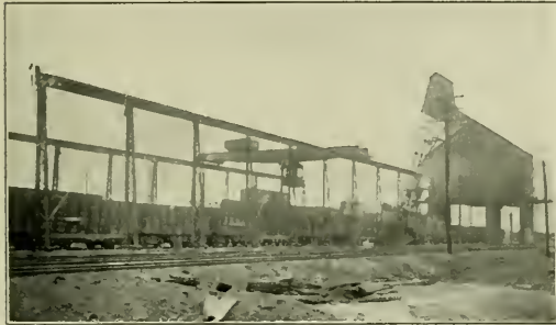
Cinder Pits and Coaling Station, Looking East.
